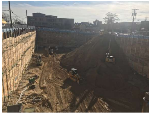
Photo 2. Example of project site with wood lagging
