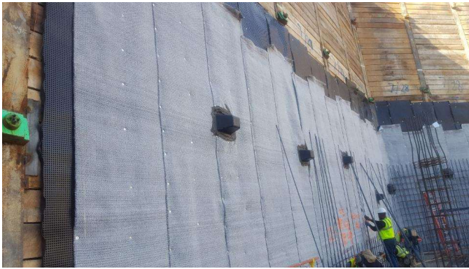
Photo 3. Example of pre-applied bentonite waterproofing onto drainage panel and wood lagging.
