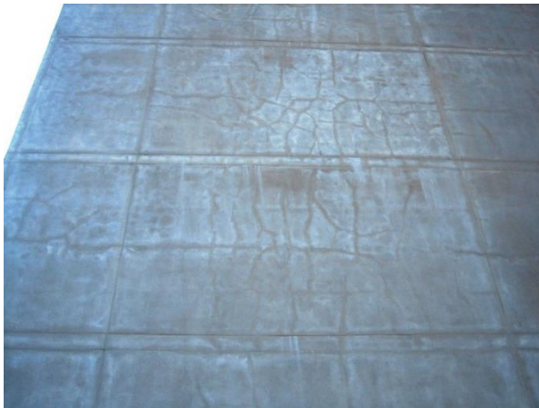
Typical map cracking due to excessive drying shrinkage
