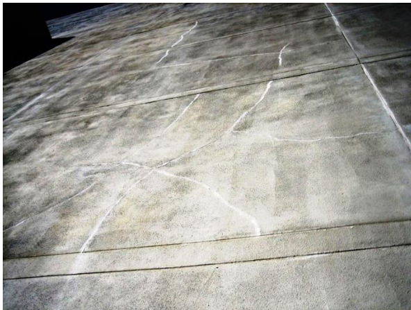
Typical map cracking due to excessive drying shrinkage
