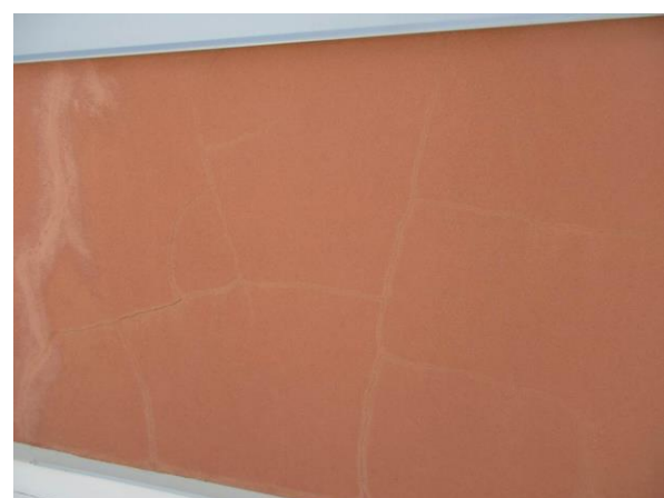
Typical map cracking due to excessive drying shrinkage
