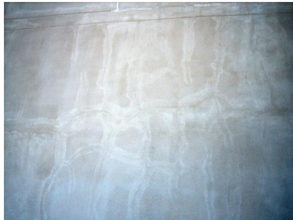
Typical map cracking due to excessive drying shrinkage
