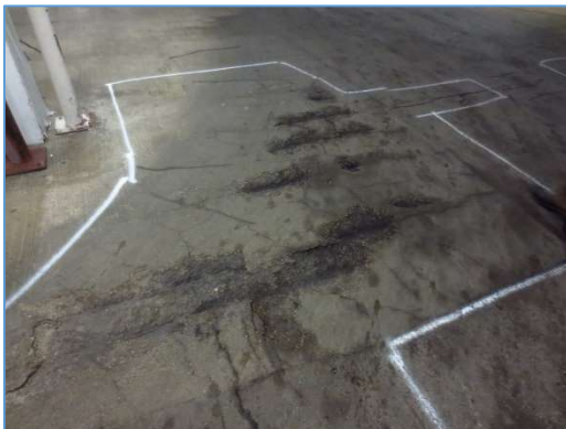
Photo 2 and 3. Example of Delamination of Concrete Surface and Soffit of Structural Slab Due to Chloride Contamination
