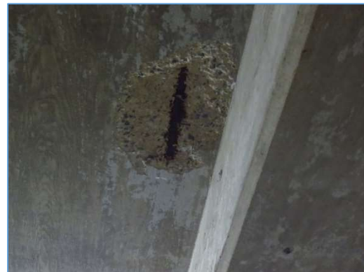
Photo 2 and 3. Example of Delamination of Concrete Surface and Soffit of Structural Slab Due to Chloride Contamination
