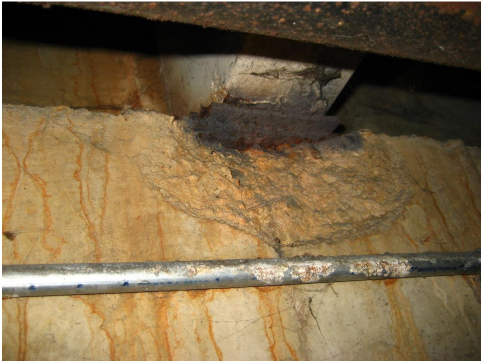
FAILED HEADER MATERIAL AND COATING AT AN EXPANSION JOINT
