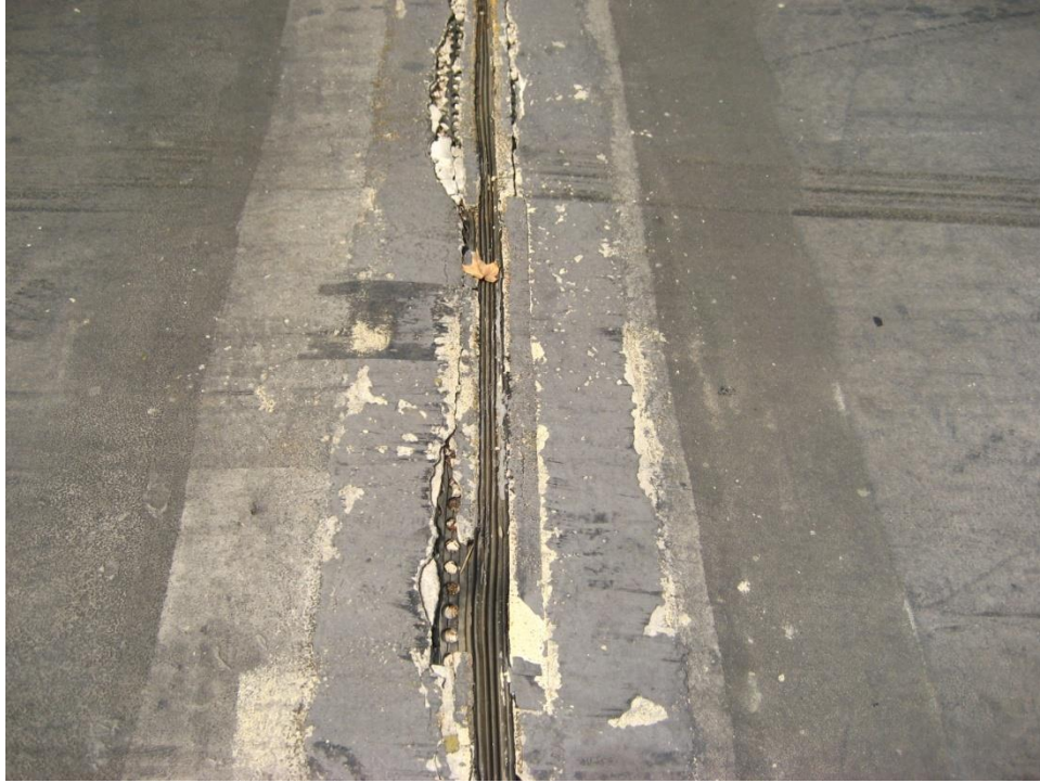
FAILED HEADER MATERIAL AND COATING AT AN EXPANSION JOINT
