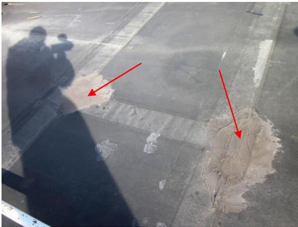
**Photo 1** – Roof repairs performed at seam failures. Seams are a typical location of roof failures.
