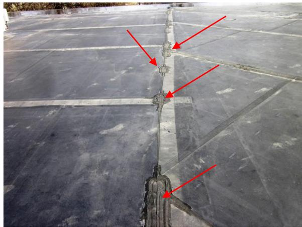
**Photo 2** – Roof repairs performed at seam failures
