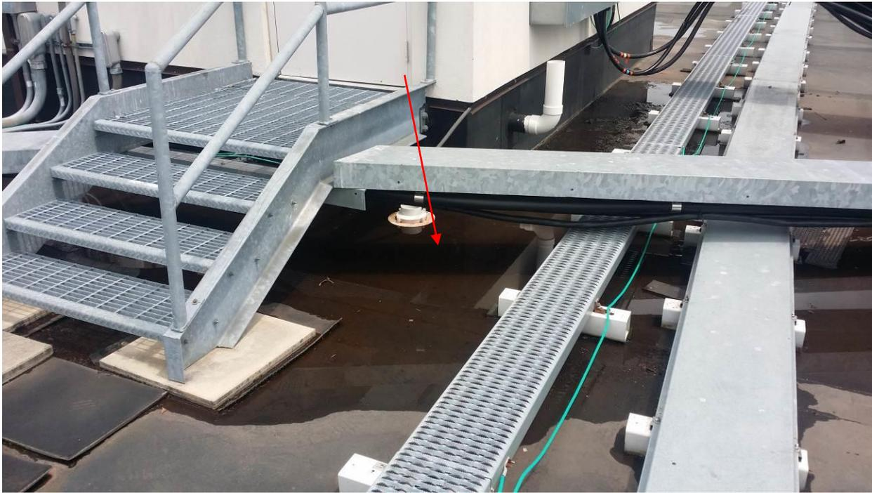
**Photo 3** – Ponding water at roof
