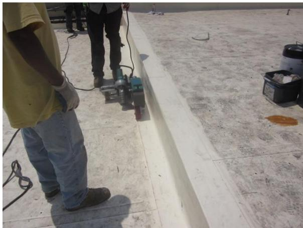
**Photo 4** – Heat welding seams in new roof
