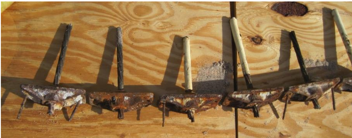
Photo 5 – Corroded PT anchors and tendons after removal from a balcony slab
