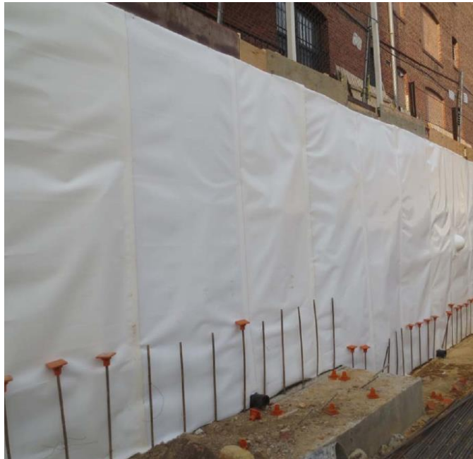
Photo 2. High Density Polyethylene Film Example against lagging
