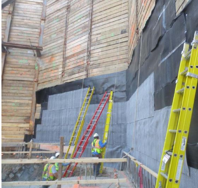
Photo 1. Bentonite System Example with Lagging
